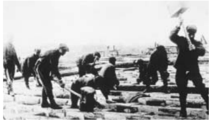
Building Lock # 1 on the White Sea Canal
